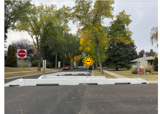
Example of Traffic Diverter Installation
