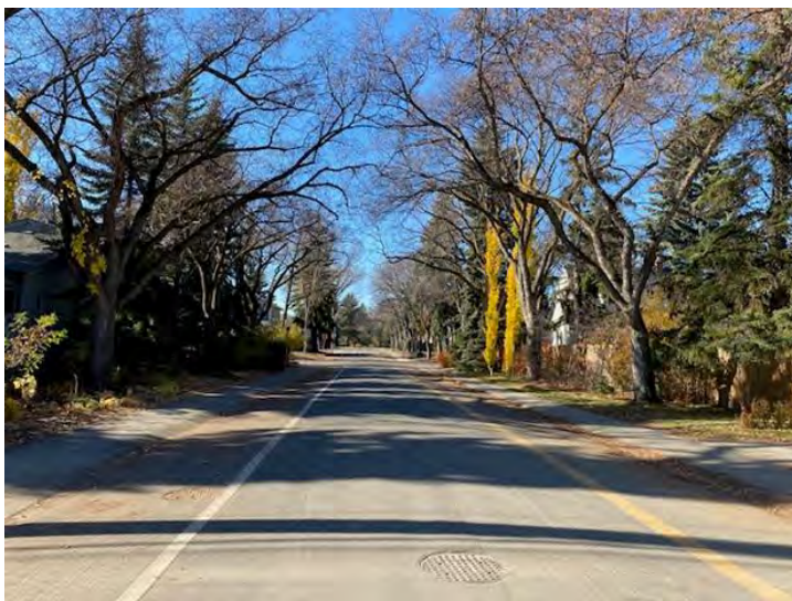
Looking west on 89 Avenue from the North-South Alley
