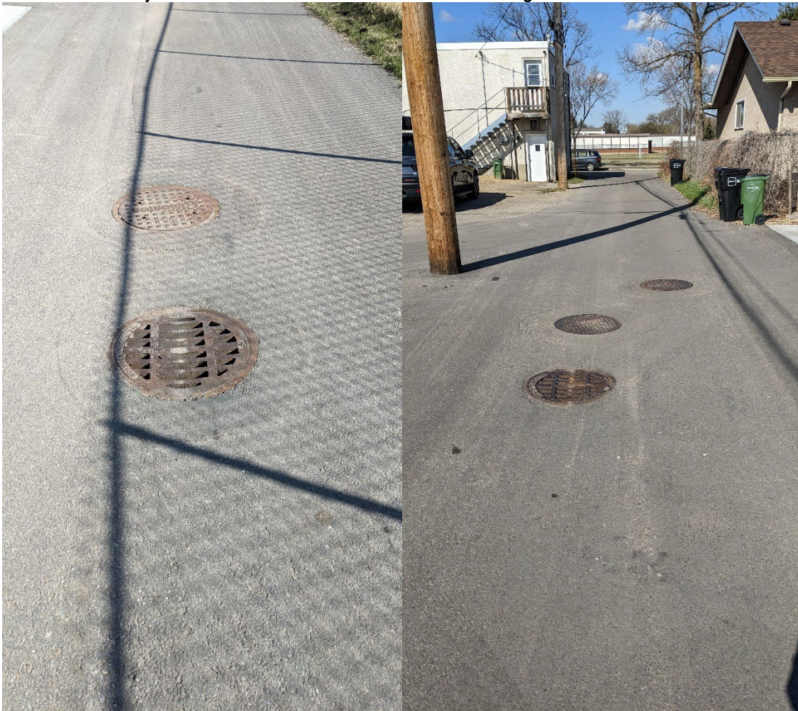
FIGURE 5. ON THE LEFT SIDE IS A VIEW FROM THE SOUTH OF THE WEST LANE, SHOWING THE TYPE 8 (F-38) CATCH BASIN, THE WEST LANE CATCH BASIN. ON THE RIGHT SIDE OF THE FIGURE IS THE VIEW FROM THE EAST SHOWING THE NORTH LANE. THIS LANE ALSO HAS A TYPE 8 (F-38) CATCH BASIN IN THE MIDDLE, THE NORTH LANE CATCH BASIN.
