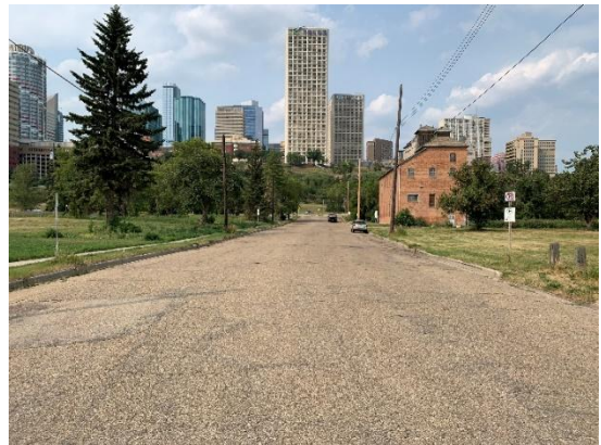
Looking North on 100 St. from North of 98 Ave.
